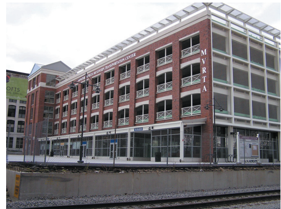
New Lawrence Station (both photos)
