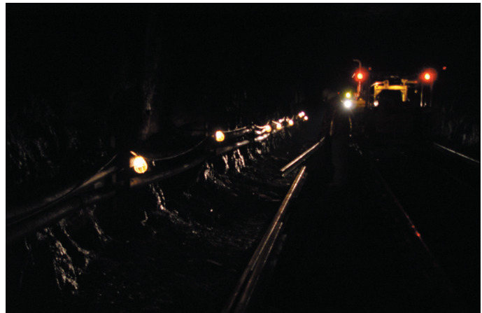
Installing Welded Rail Deep in the Tunnel Photo by Phil Corder
